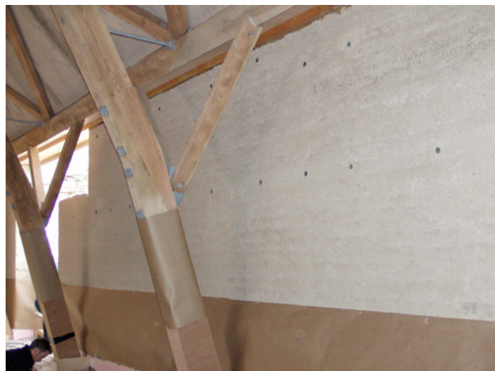
Figure 10.11: Sheepdrove Organic Farm, Berkshire
